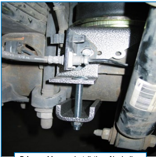
Drivers side rear. Installation of brake line.
