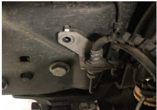
Figure 2B: OE Brake Line Bracket, Bolt Removed
